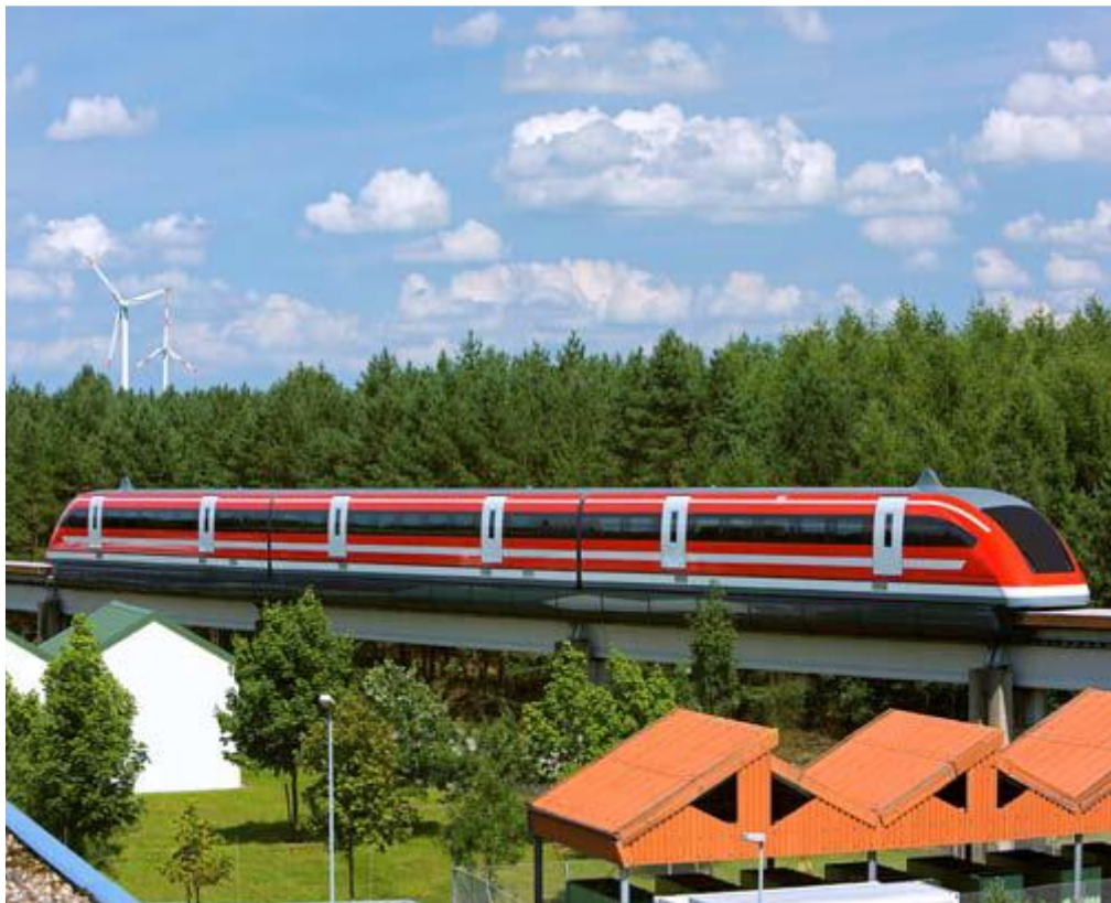
Figure 10 - TR09 in operation on TVE
