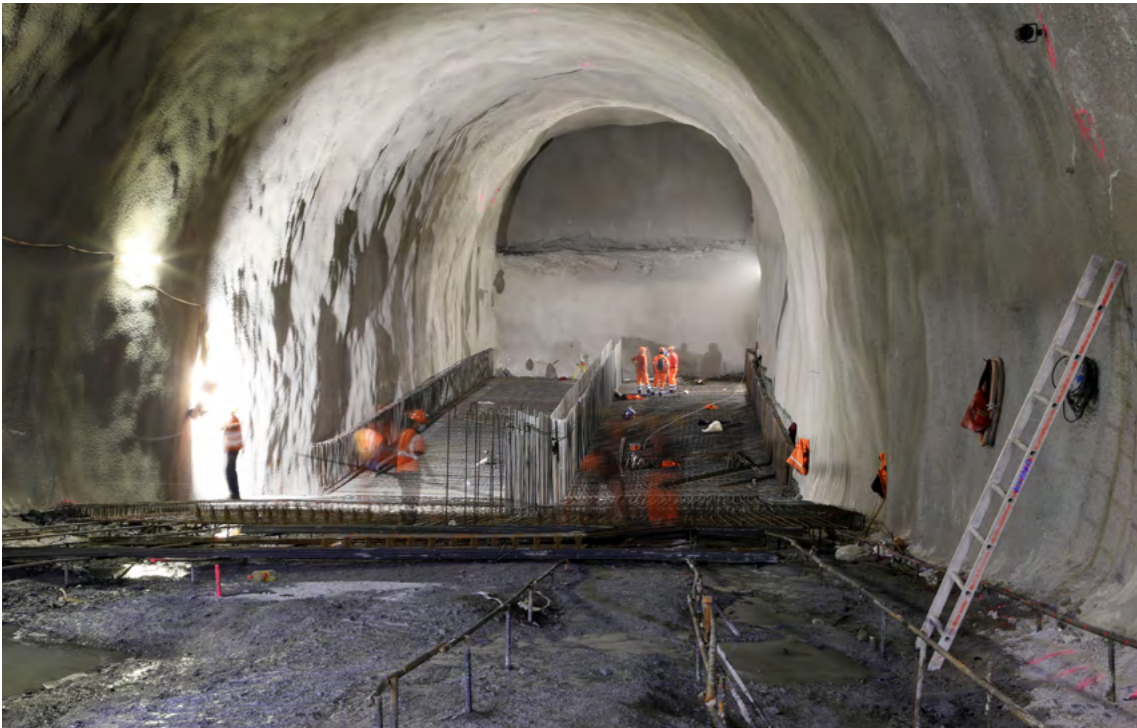
After the incident in the Lötschberg Tunnel the soil and walls of the cavern were reinforced. More information can be found on the BLS Website .
