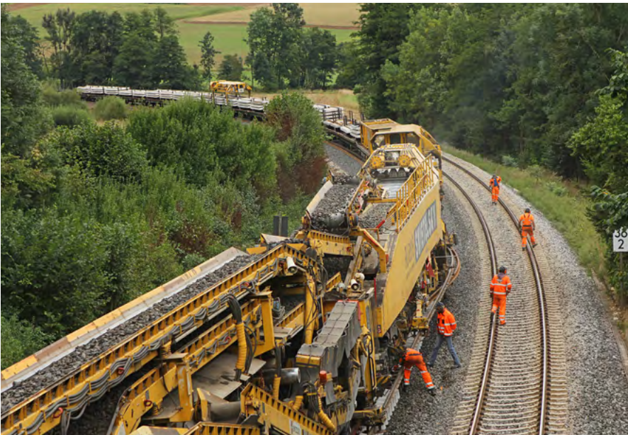
High output maintenance work with a track renewal machine on the German network.
