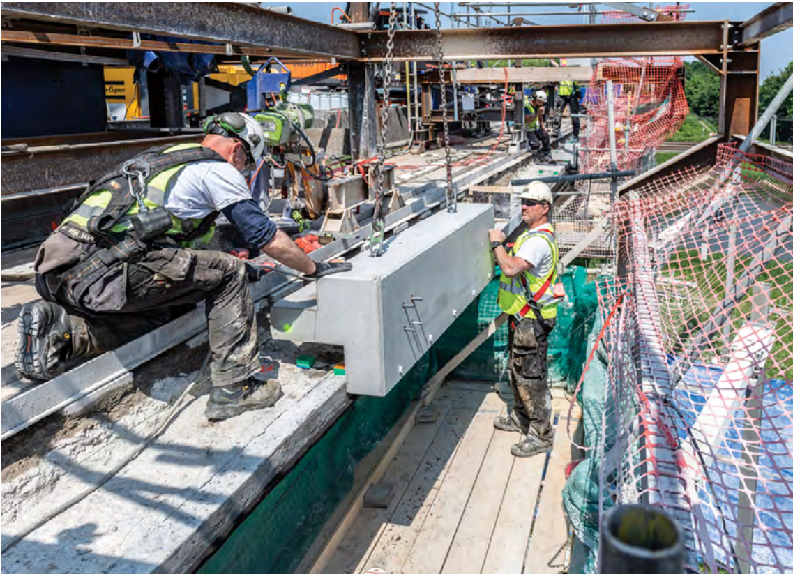
Replacement of bridge sections on the Munnikensteeg viaduct near Kijfhoek.
